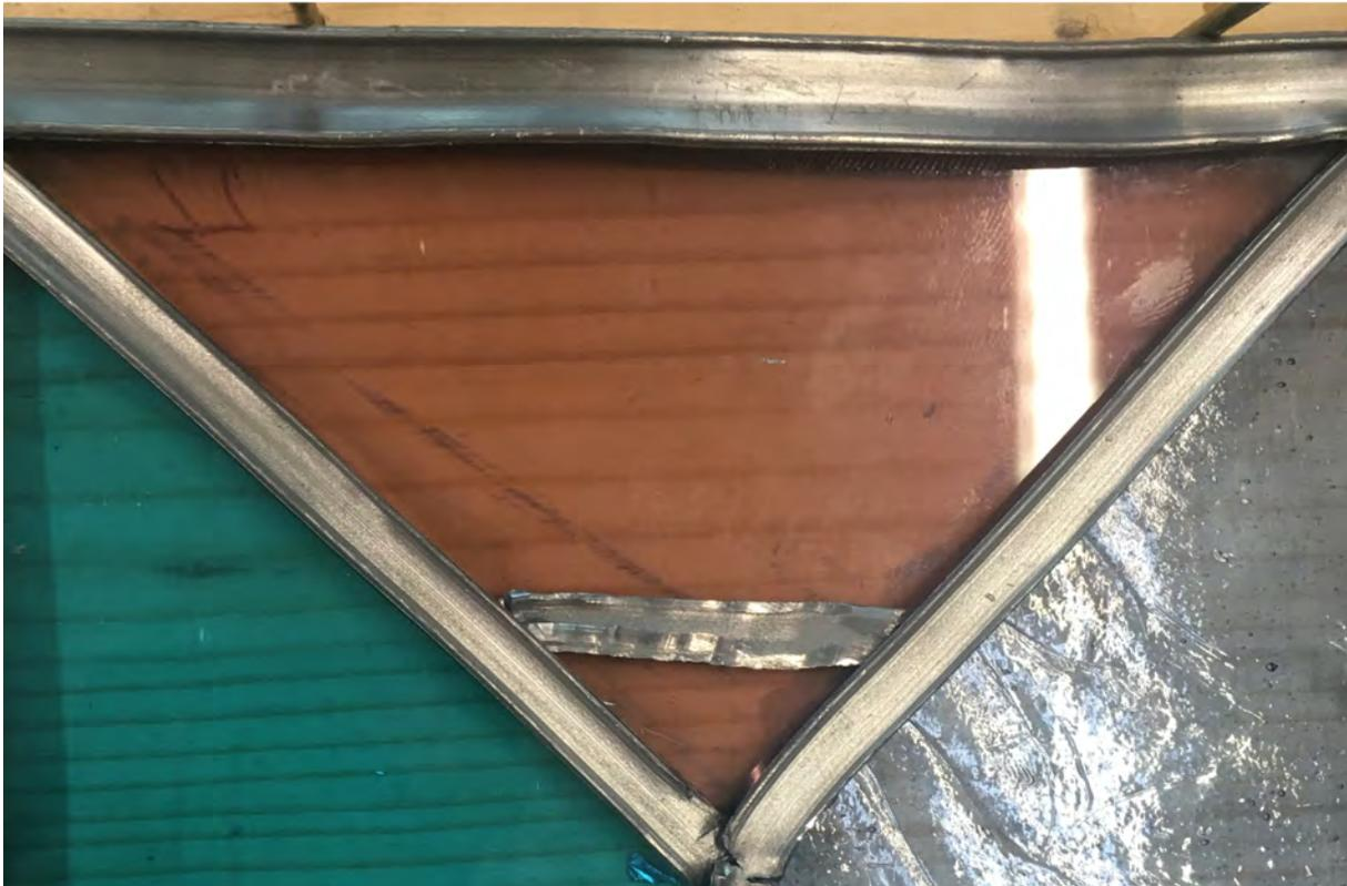
Figure 47: Top of the lead came placed on the crack.
