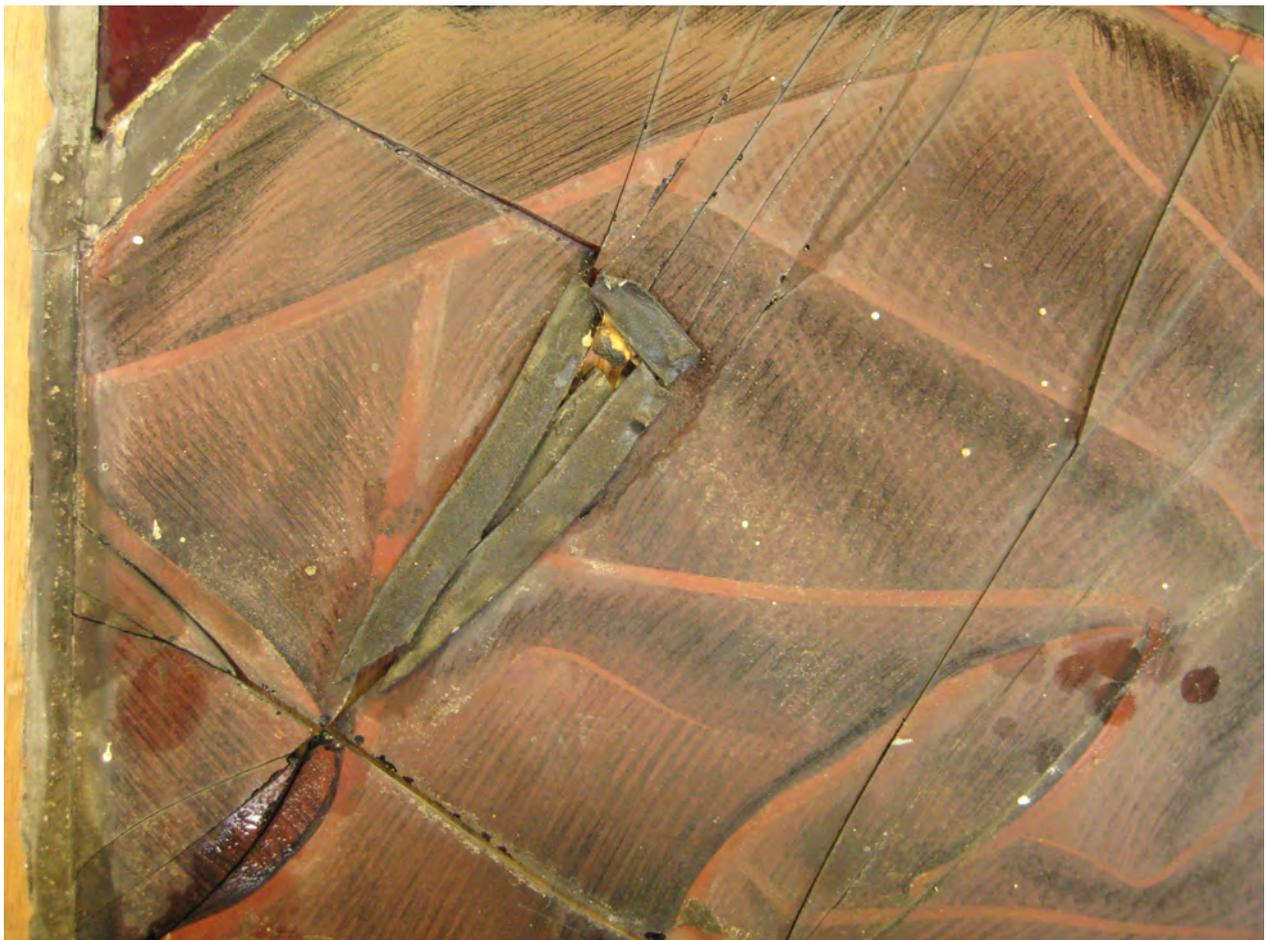
*Figure 36: Example of re-leading, where the lead came is just inserted in the break and not even soldered. Image provided by M. de Caluwé, 2022.*
