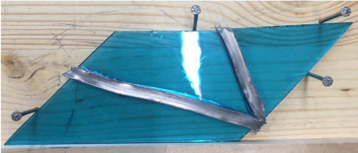
Figure 41: The damaged piece with the lead came measured and cut to size. Image by L.Ristal, 2022.
