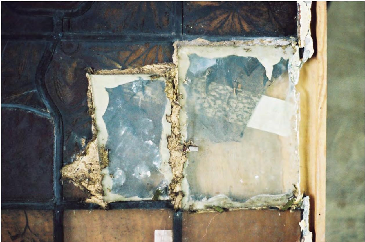
*Figure 31: Example of a putty edge bond. Image provided by M. de Caluwé, 2022.*
