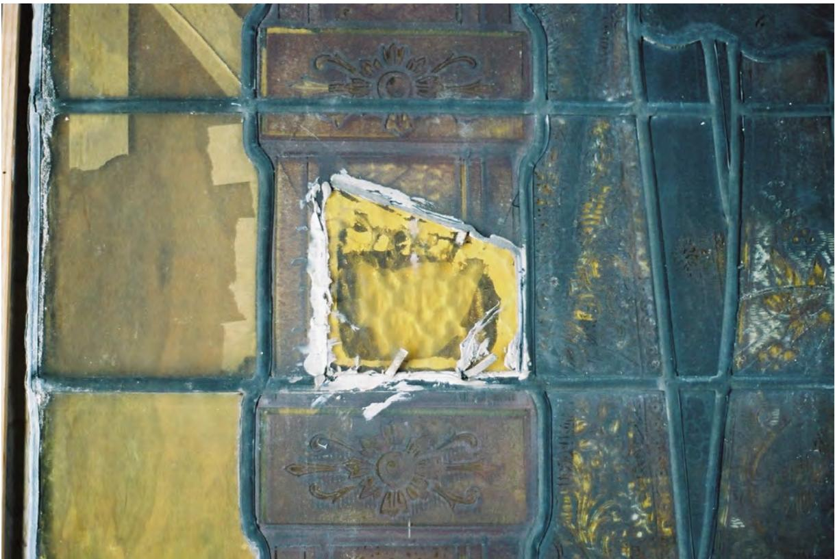
Figure 32: Example of a putty edge bond. Image provided by M. de Caluwé, 2022.
