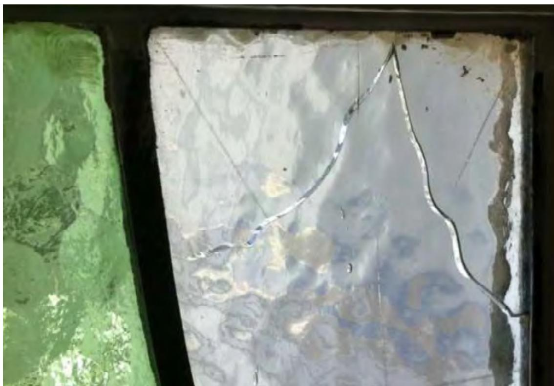
Figure 28: Heat crack. Image by S. Hardingham, *An Analysis of Stained Glass Fabric Specific to Conservation Assessment*, p 10.
