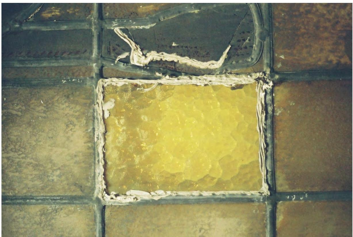
Figure 33: Example of a putty edge bond. Image provided by M. de Caluwé, 2022.
