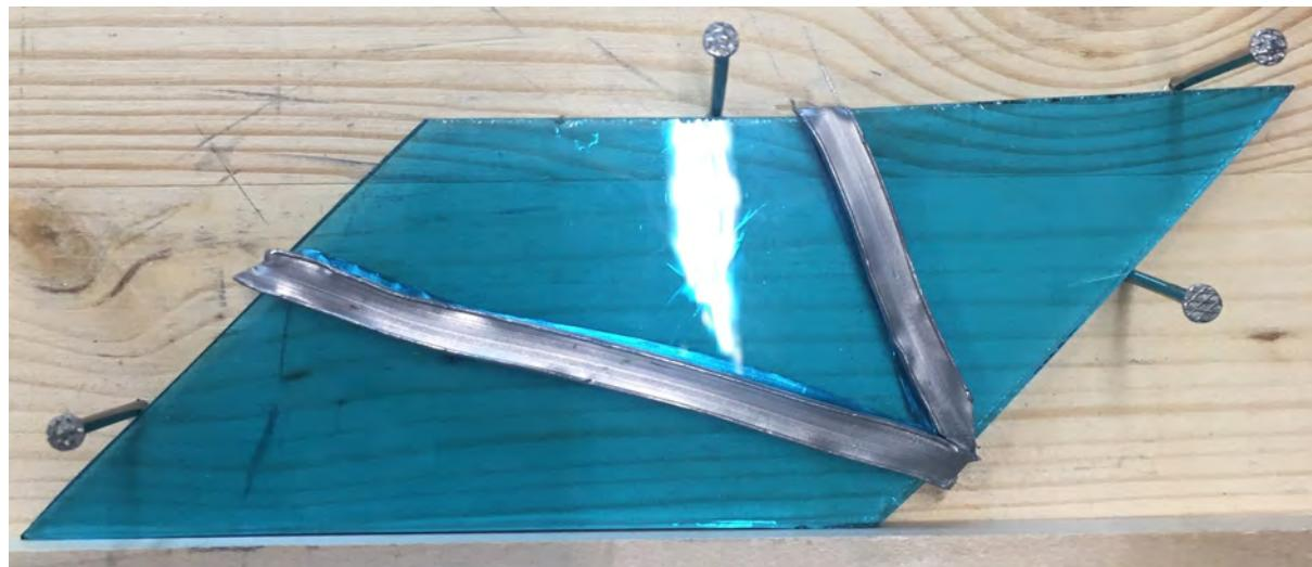
Figure 41: The damaged piece with the lead cames measured and cut to size. Image by L.Ristal, 2022.
