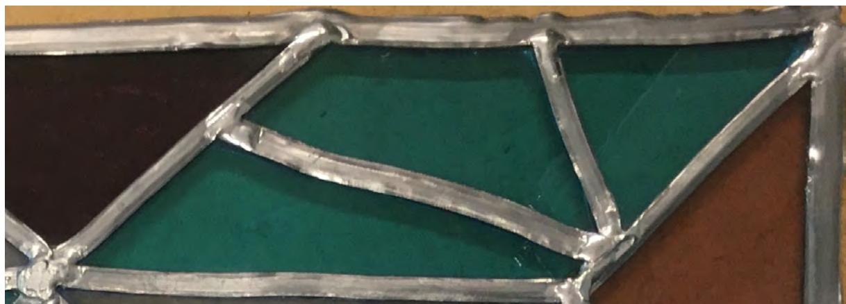
Figure 43: The finished lead repair in the panel. Image by L.Ristal, 2022.
