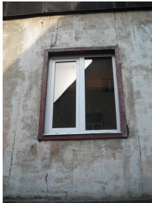
35. Vasak W-1.korruse aken (PVC).
