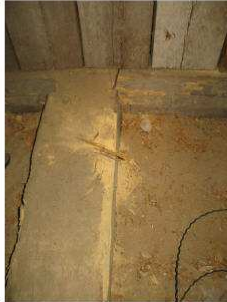
Fig. 29. Roof construction (right side)
