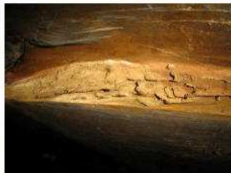
Fig. 7. Old damage by HB
