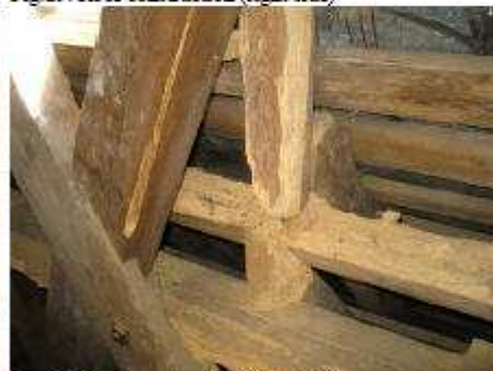
Fig. 31. Roof construction (right side)
