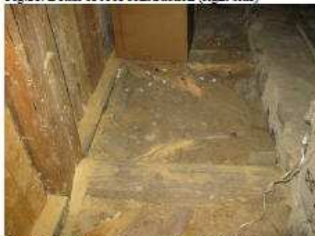
Fig. 30. Detail of roof construction (right side)
