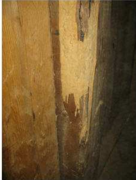
Fig. 28. Detail of roof construction (right side)
