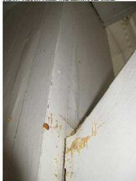
Fig.17. Loose surface and frass
