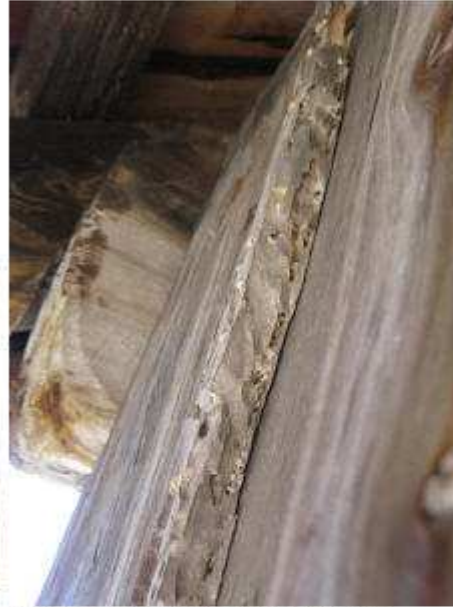
Fig. 9. Detail of active HB attack in panelling
