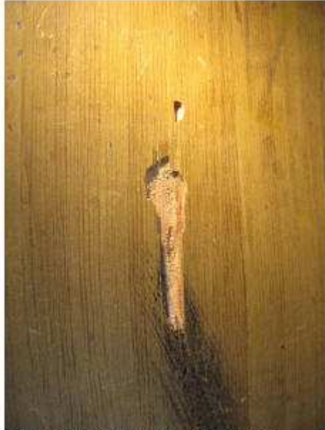
Fig.14. Detail of bench with broken-off surface
