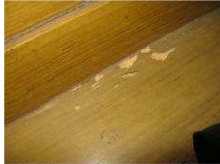
Fig.11. Detail of active HB attack in bench
