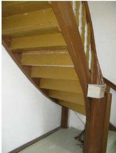
Fig.20. Stair case to gallery
