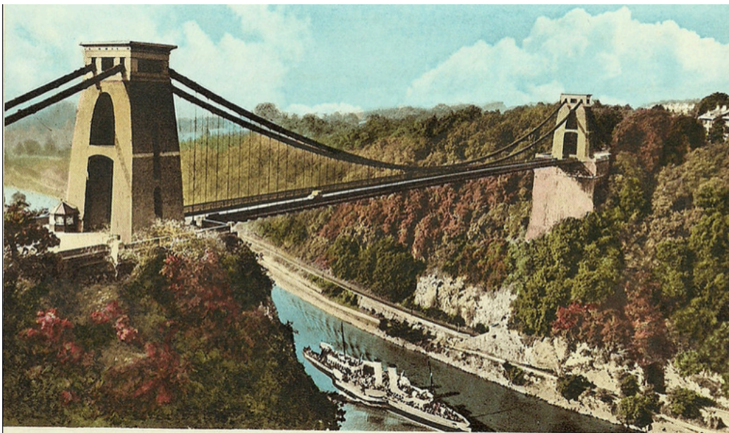
5. Clifton Suspension Bridge.
