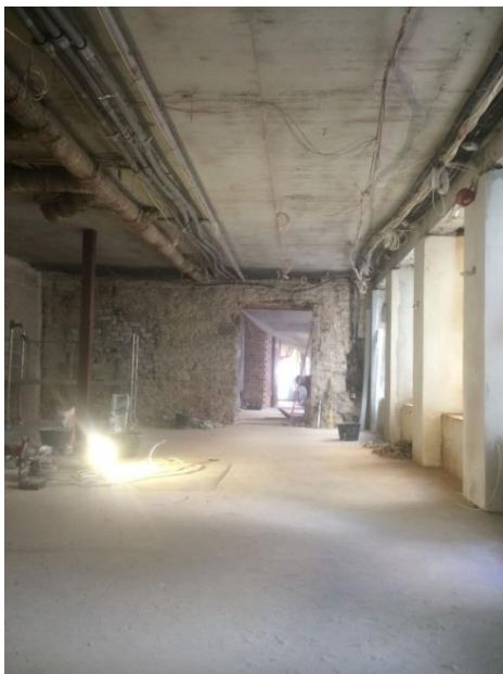
Sama ruum remondi ajal 2016. 53 Betoon.
