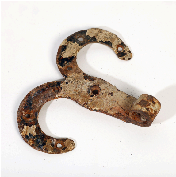
Joonis 64. Sepisdetail: oinasarv-hing.
