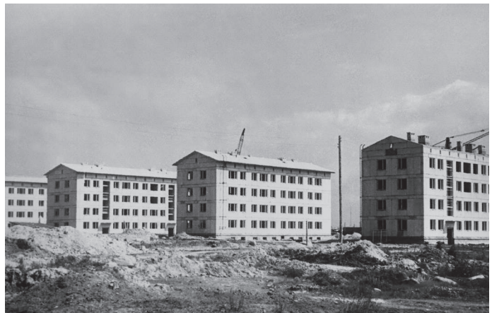
4.14: Esimesed silikaltsiididetailidest suurkorterelamud ehitati Pelguranda. The first large apartment blocks made using silicalcite were built in Pelgurand.
