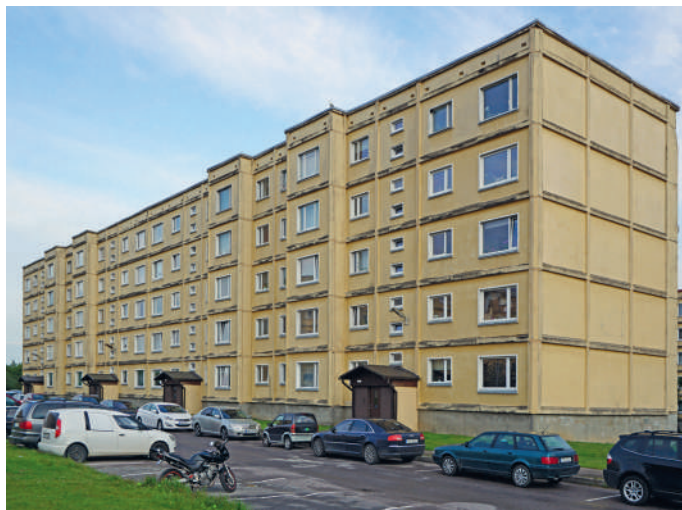
5.12: Tartu Elamuehituskombinaadi kolmekihilistest ribelistest seinapaneelidest kortermaja ehk nn „vahvelmaja” Tartus Annelinnas. Apartment building in Annelinn, or “waffle houses” as they were referred to, were made from triple-layered ribbed wall panels made by the Tartu Housing Construction Plant.
