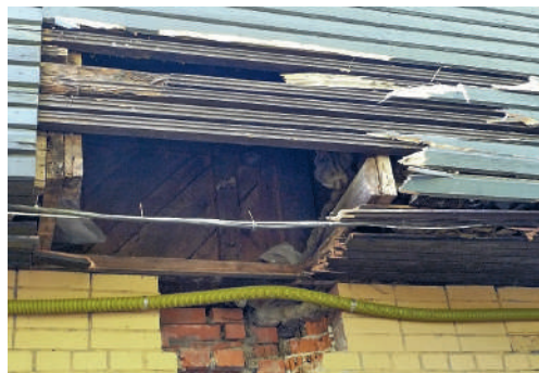
1.03: Kohviku Tuljak uurimistöödel leiti hilisema laudise alt osaliselt säilinud algne karniisilaudis. During restoration of Tuljak café, partially intact original cladding emerged from under cladding that had been applied later.
