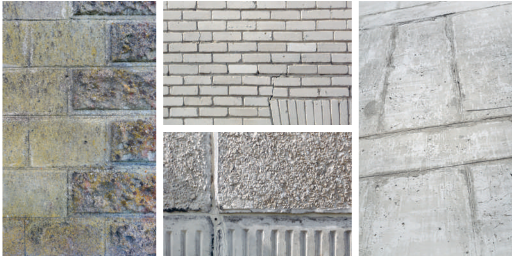
S.03: Betoonkivid, silikaattellised, silikaltsiidist suurplokid ja raudbetoonist suurpaneelid on tugevalt kujundanud Eesti 20. sajandi arhitektuuripilti. Concrete blocks, calcium silicate bricks, silicalcite blocks and prefab reinforced concrete wall panels have played a significant role in shaping Estonian architecture of the 20th century.
