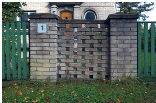
3.53: Tellistest laotud piludega ilupiire. Decorative brick fence.
