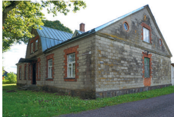
2.04: Lehtse hoiu-laenuühisuse majas (1914) on betoonkivi kombineeritud punase tellisega. Lehtse Savings and Loan Society Building (1914) has concrete blocks used in combination with red bricks.
