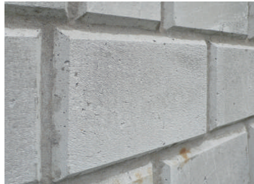
2.36: Faasitud servadega tuhaplokkid abihoone seinas. Fly ash blocks with bevelled edges in an outbuilding wall.
