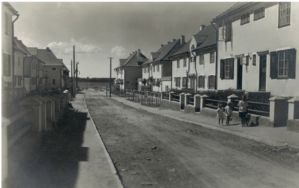
2.20: Elamukooperatiivi Oma Kolle elamud (1923–1926) Tallinnas Pelgulinnas olid moodsad ka seinakonstruktsioonilt, milles kasutati betoonist õõneskive ja T-kujulisi betoonkive. Housing cooperative "Oma Kolle" houses (1923–1926) in Pelgulinn, Tallinn were also considered modern for their wall construction, which used hollow and T-shaped concrete blocks.
