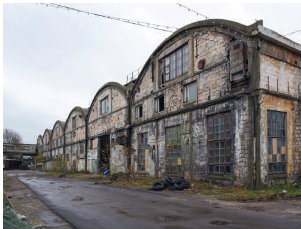
2.05: Bekkeri laevaehitustehase sepikojahoone (1913) seinad on ehitatud suureformaadilistest betoonkividest. The walls of the blacksmithing workshop at the Bekker shipyard (1913) are made from large concrete blocks.
