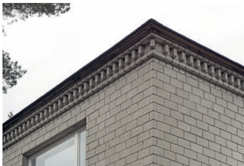
3.52: Hammaskarniis oli nõukogude perioodi individuaalmajade dekoreerimisel sage võtte. Saw-tooth cornices were a common decorative device on single-family homes during the Soviet period.
