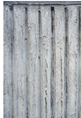
5.29: Lohaka viimistlusega soklipaneel. Basement level panel with sloppily stamped details.
