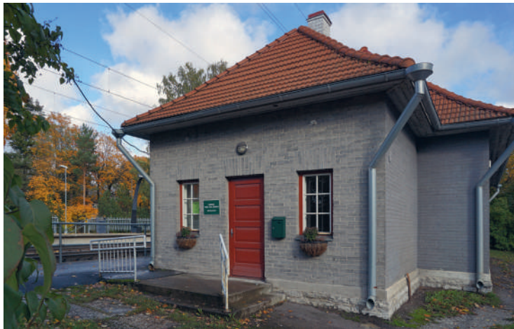
3.24: Rahumäe jaamahoone (1930) on ehitatud krohvimata tuhttellistest. Rahumäe railway station (1930) built using unrendered fly ash bricks.
