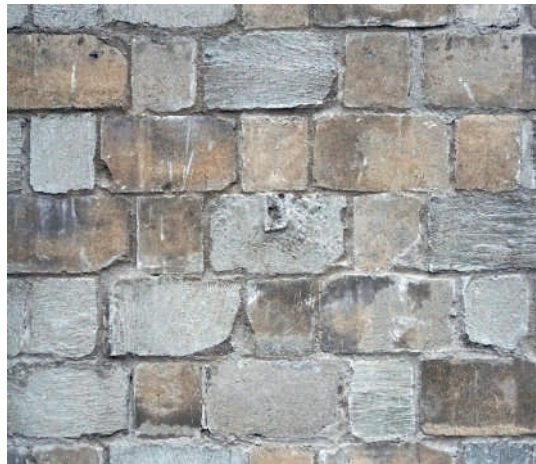
2.38: Tallinna vesilennukite angaari betoonkividest sein pärast restaureerimist. Concrete block wall at Tallinn's seaplane harbour after restoration.
