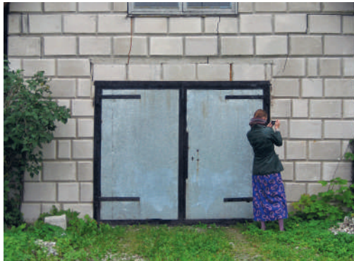
2.36: Faasitud servadega tuhaplokkid abihoone seinas. Fly ash blocks with bevelled edges in an outbuilding wall.
