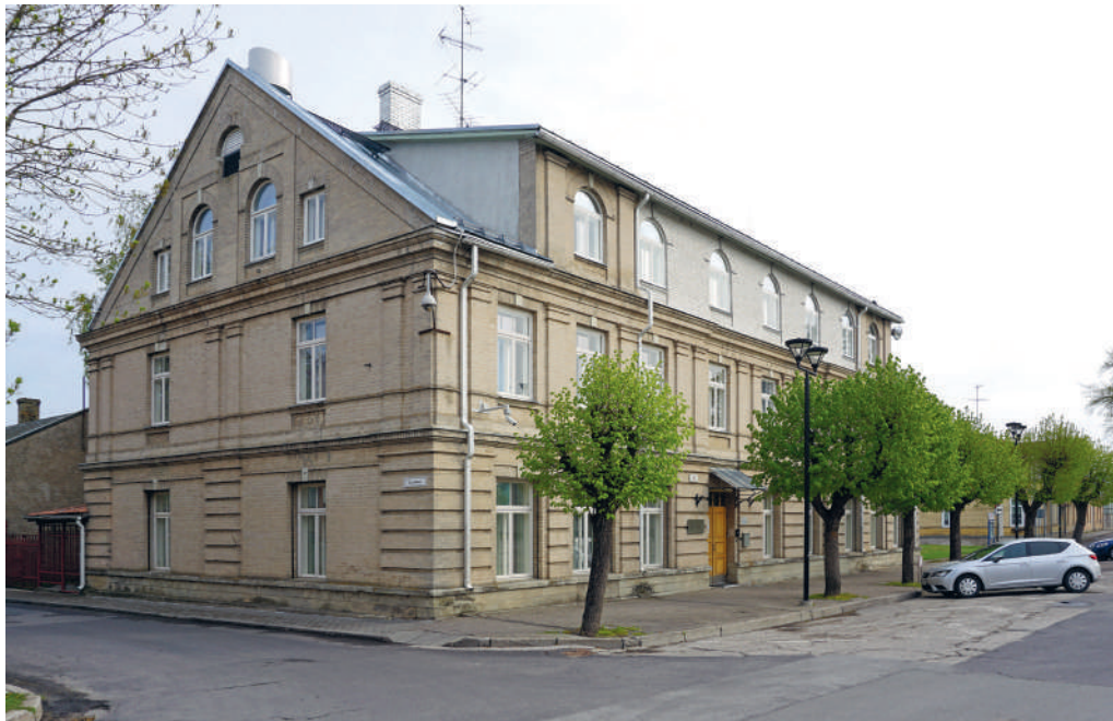
3.03: Siegfeldti ärimaja Haapsalus Lossiplats 4 (1912) on ehitatud oma aja kohta erandlikult krohvimata silikaattelistest. The Siegfeldt commercial building at 4 Lossiplats, Haapsalu (1912) was built using unrendered silicate bricks, which was unusual at that time.
