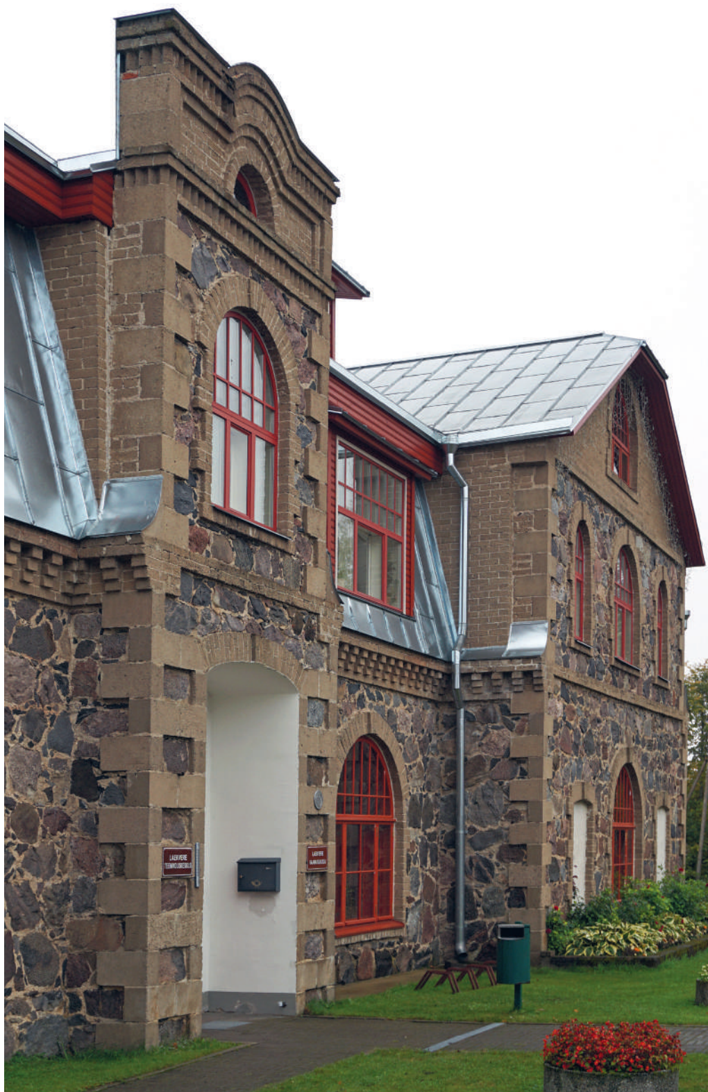
2.26: Endine meierei hoone (1931) on osa Laekvere keskuse omanäolisest hoonestusest, milles kohtuvad maakivi ja betoonkivid. This former dairy (1931) is part of the distinctive buildings in Laekvere where natural stone meets concrete blocks.
