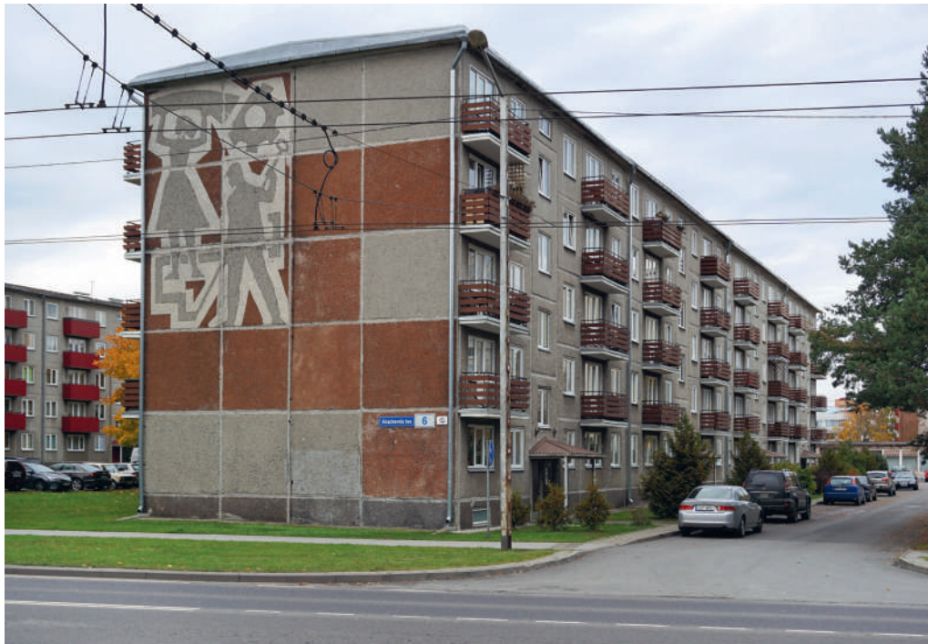
5.42: Elamu Tallinnas Akadeemia tee 6 on üks väheseid paneelmaju, millel on taastatud algsed röödupiirded. The apartment building at 6 Akadeemia tee in Tallinn is one of the few prefab buildings where the original balcony railings have been restored.
