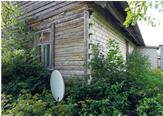
3.44: Silikaattellist kasutati sageli vanemate hoonete renoveerimisel. Silikaatvoodriga rehemaja Saaremaal. Silicate bricks were often used in the renovation of older buildings. Silicate lined barn-dwelling in Saaremaa.
