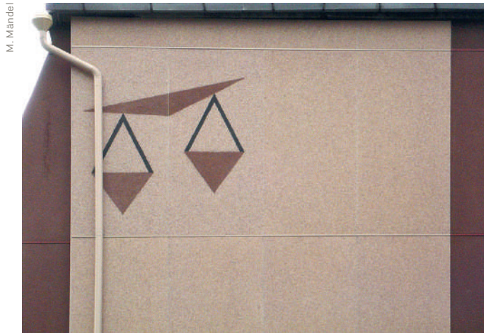
5.43: Hoone renoveerimisel on soojustuse alla jäänud monumentaalpannoo lihtsustatult kantud soojustuse pinnale. The large mural designs, covered by insulation during renovation, have been transcribed in a simplified form onto the surface of the insulation.
