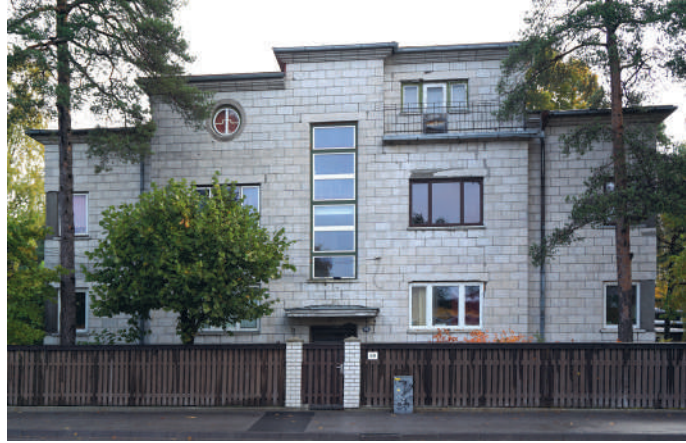
2.32: Kortermaja Tallinnas Männiku tee 59 [K. Tarvas] on ehitatud heledatest Toomanni kividest. This apartment building at 59 Männiku tee, Tallinn [K. Tarvas] is made from pale Toomann blocks.
