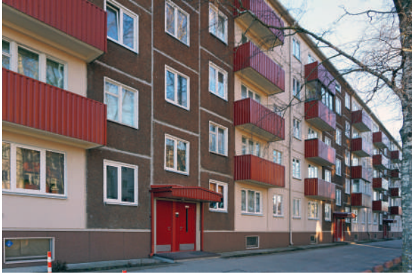
5.21: Karjamaa asumi paneelmajal on kombineeritud värvitud sileda-pinnalisi paneele ja punaka graniitkivikillustikuga kaetud paneele. Prefab apartment building in Karjamaa has a combination of smooth panels and panels coated with reddish granite grit.
