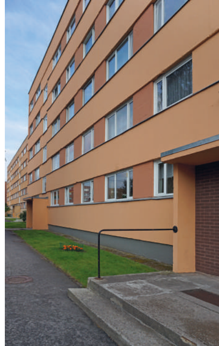
5.08: Tartu Elamuehituskombinaadi gaaskukeroon-seina-paneelidest „triibuline” maja Annelinnas. “Striped” buildings in Annelinn made from oil shale ash concrete wall panels made at the Tartu Housing Construction Plant.
