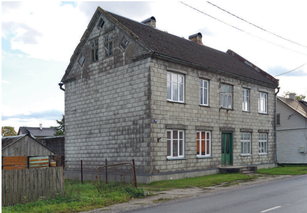
2.34: Arnold Toomanni elamu Tapal Ambla mnt 23 on valminud samal õuel toodetud kividest ning on Toomanni toodangu kasutuse üks paremaid näiteid. Arnold Toomann's home at 23 Ambla maantee, Tapa was built using the blocks that were made in his yard and is one of the best examples of the use of Toomann's products.
