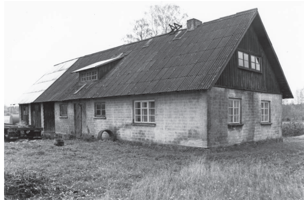
2.24: Palju kasutati nopsaseina asundustalude juures. The Nopsa wall was often used to build settler farmhouses.
