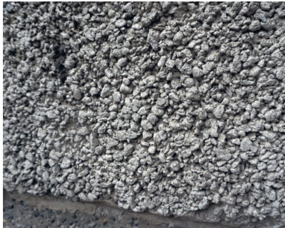
5.20: Lähivaade Mustamäe maja seinapaneelist, kus tsemendijääke pole maha pestud. Close-up of a wall panel on a building in Mustamäe where the excess cement has not been washed off.
