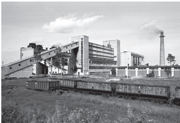
5.09: Oru turbakombinaat (1963, Ü. Ilves) oli esimene gaaskukeroon-paneelidest tööstushoone. Oru Peat Works (1963, Ü. Ilves) was the first factory building to be made of oil shale ash concrete panels.
