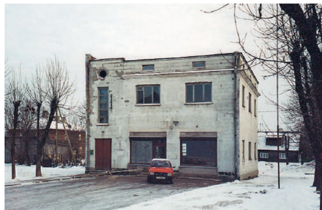
2.33: Heledad ja siledad Toomanni kivid sobisid hästi funktsionalistliku arhitektuuriga. Bussiliinide pidaja A. Pärna elamu Tapal [1938, lammutatud]. The light coloured smooth Toomann blocks were well suited to Functionalist architecture. Home of bus company owner A. Pärn in Tapa [1938, demolished].
