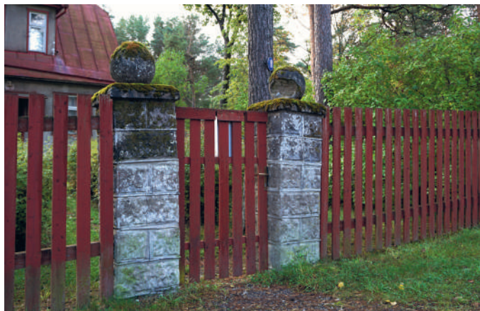
2.29: Betoonkividest väravapostid olid Nõmmel tavalised. Concrete block gateposts are common in the suburb of Nõmme.
