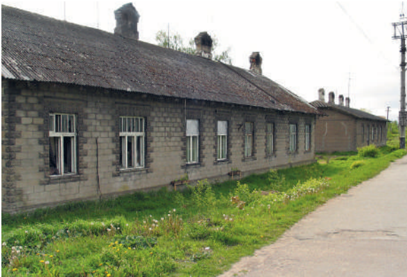
2.03: Tööliselamud Kehra jaamas (1910. aastad) muudab ilmekamaks klombitud looduskivi imiteerivate betoonkivide kasutamine hariliku siledapinnalise betoonkivi kõrval. The barracks at Kehra railway station (1910s) are enhanced by the use of concrete blocks rusticated in imitation of natural stone alongside ordinary, smooth concrete blocks.
